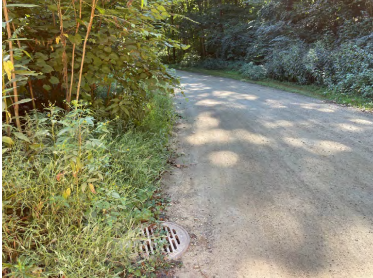
Photo 10: Stormwater inlet on River Front Drive draining to CMP outfall.
