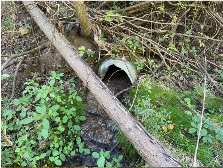
Photo 9: Third CMP outfall under River Front Drive draining from north slope of Red Bud Trail into the wetland on south side of the River Front Drive.
