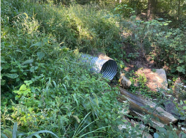
Photo 7: Second CMP outfall draining from north of River Front Drive into the wetland on the south side of the road.
